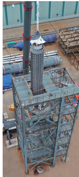
薄膜蒸发器组装试运转 Assembly and Trial Operation of Thin Film Evaporators
